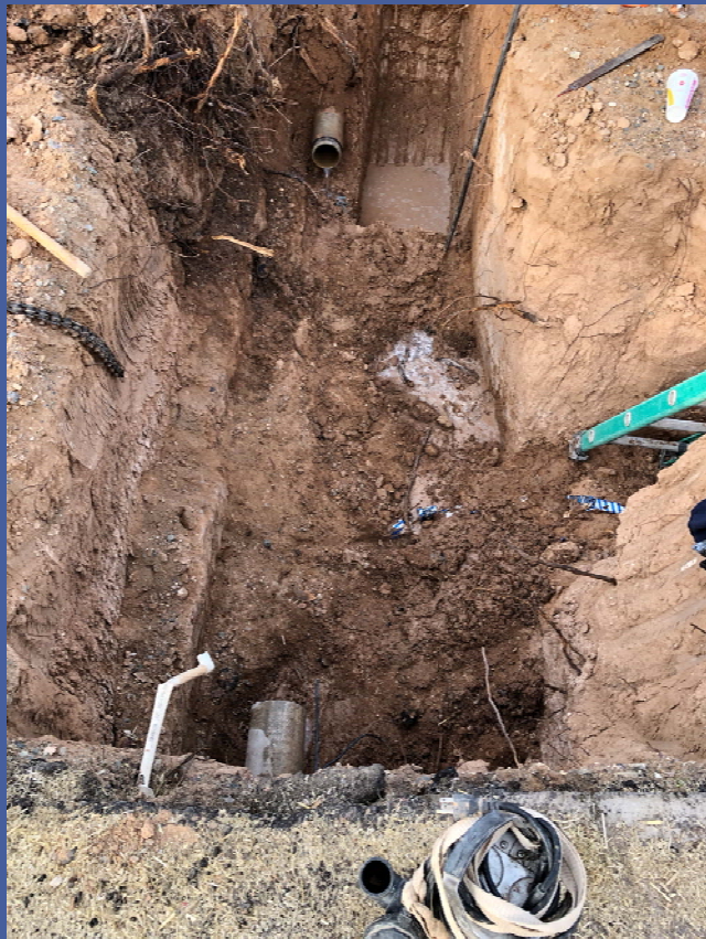
Remove Section of Pipe for New Hydrant
